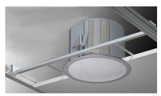
**Figure 6.** Position of loudspeaker relative to bridge support rails during installation Align the flat sides of the can with the tile support rails
